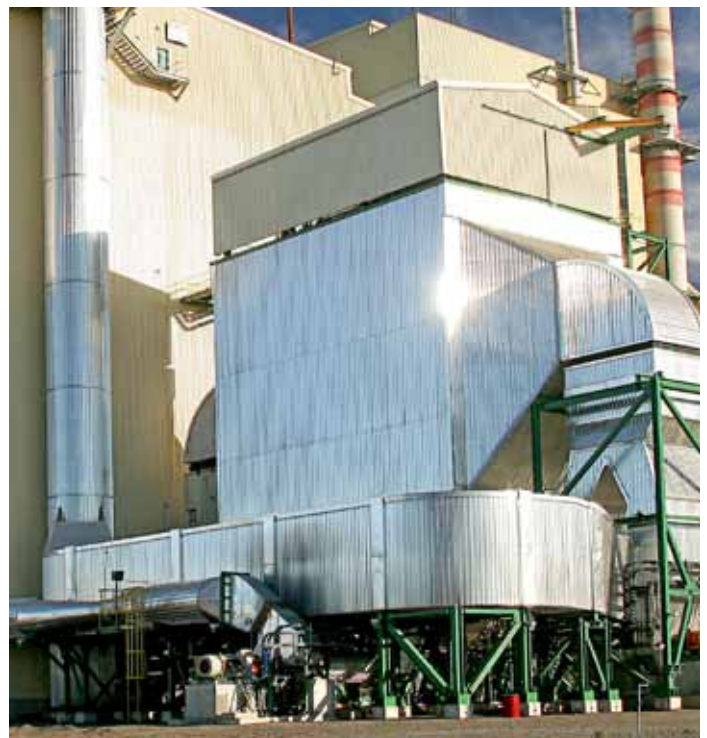
> Particle electrostatic precipitator of the new biomass boiler at the Santa Fe Pulp Mill.
