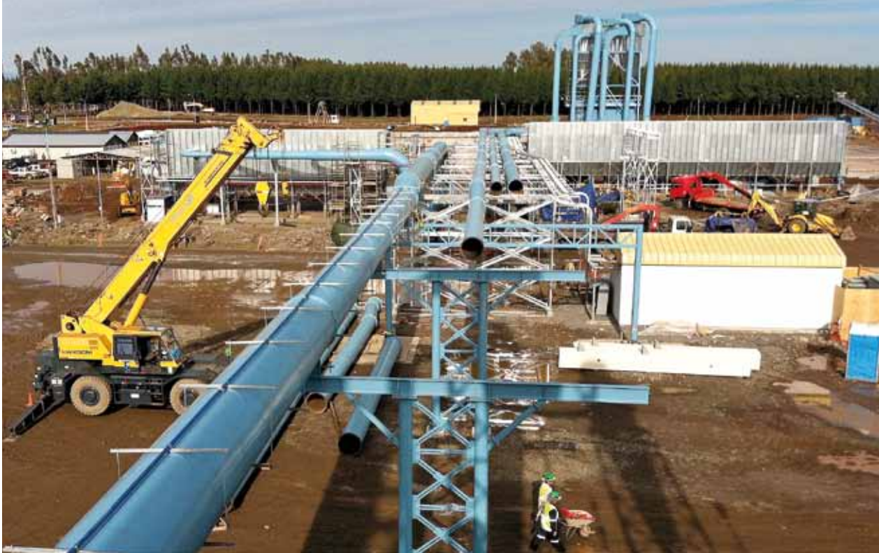
> Industrial contractors assembling the extraction system, filtering and particle handling of wood chips and sawdust from sanding machines, as part of expansion works at the Plywood Plant, located in Mininco, district of Collipulli, Araucanía Region.
