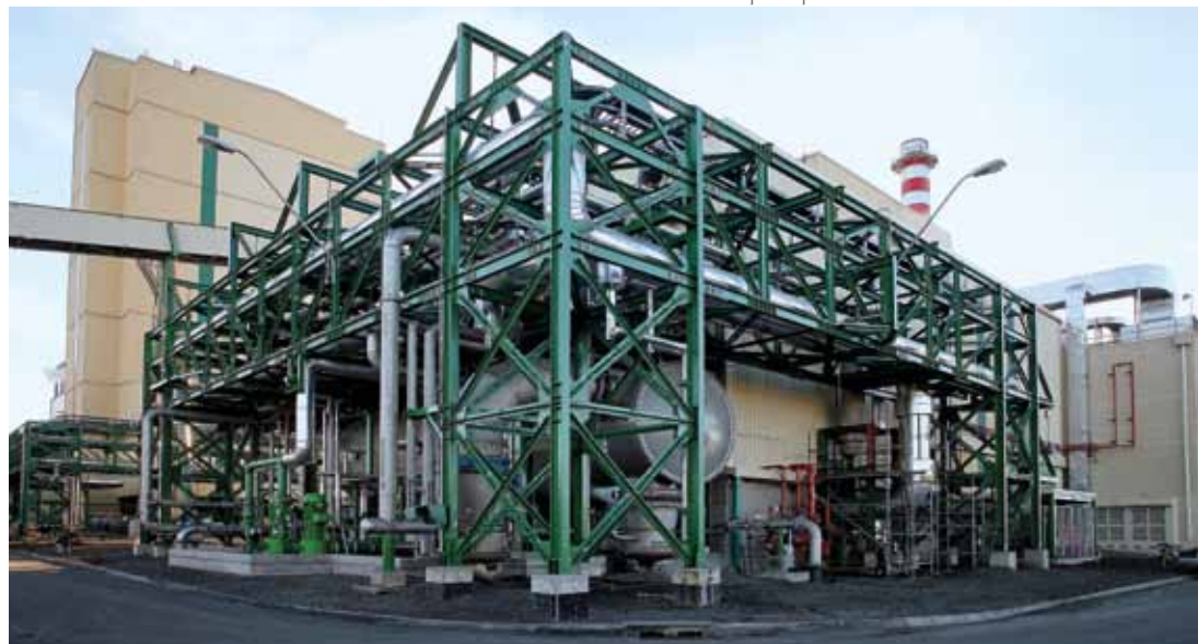
> Biomass boiler equipped with particle electrostatic precipitator.
