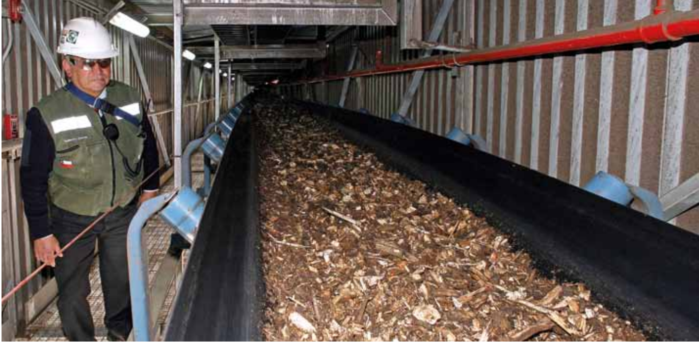
> Biomass mixture transported by the conveyor belt to the boiler.
