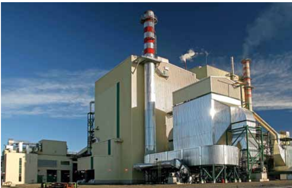
> Biomass boiler equipped with particle electrostatic precipitator.
