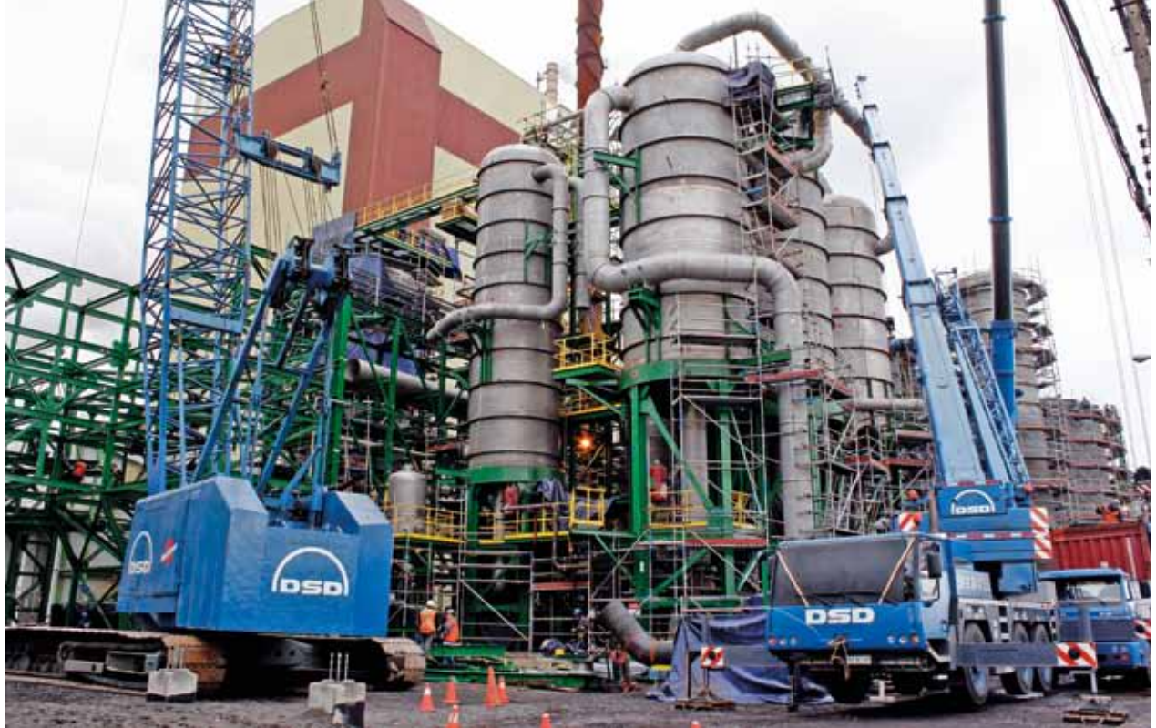
Industrial assembly contractors working on the project of modernization of the Laja pulp mill.
