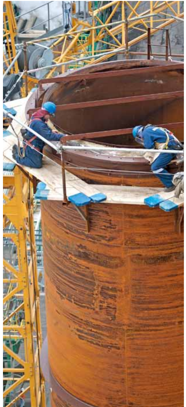
> Erection of the new recovery boiler exhaust stack at the Laja Pulp Mill.
