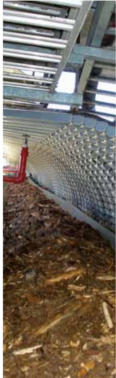
> Biomass being transported to the Pacific Pulp Mill boiler.
