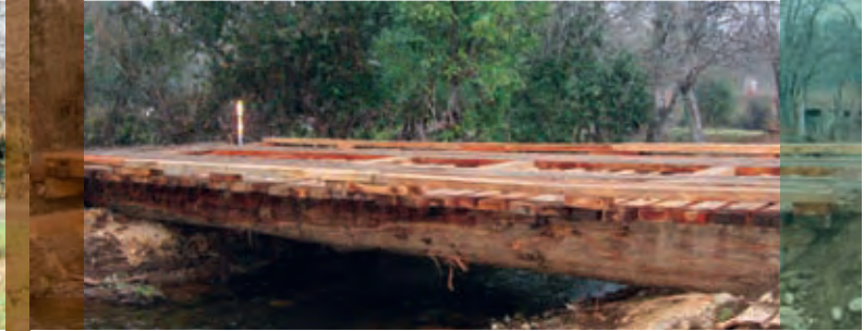
Construction of new local wood bridge in La Frutilla sector, district of Loncoche, Region of Araucanía that benefitted 30 people of the locality of Collimallín. Above, the new, more resistant bridge; and to the left, the old and weakened bridge.
