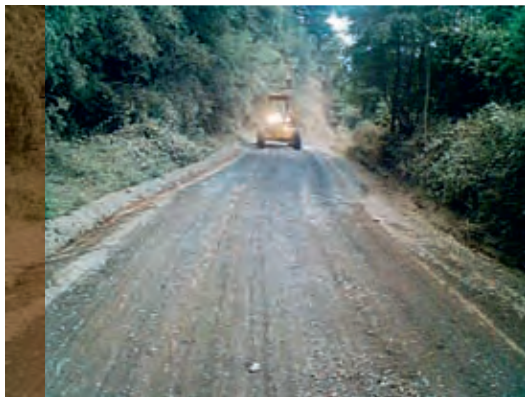
Improvement of paving with crushed, compacted material in the local public road from the El Piulo crossing up to Quilahueque hill, a distance of 3,5 kilometers in the Loncopangue sector, benefitting 560 people of the district of Quilaco, Bío-Bío Region.
