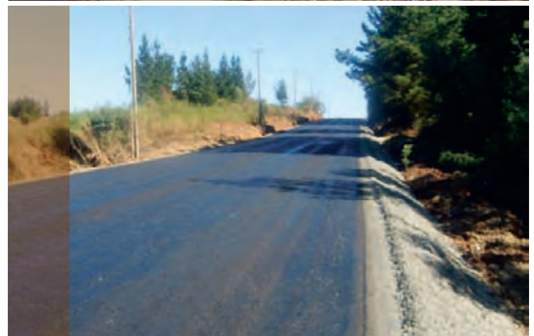
Asphalt paving, 7 meters wide, with stabilized shoulders; paving executed by Forestal Mininco in the sector of the Mulchén bypass towards El Morro, Mulchén district, Bío-Bío Region.
