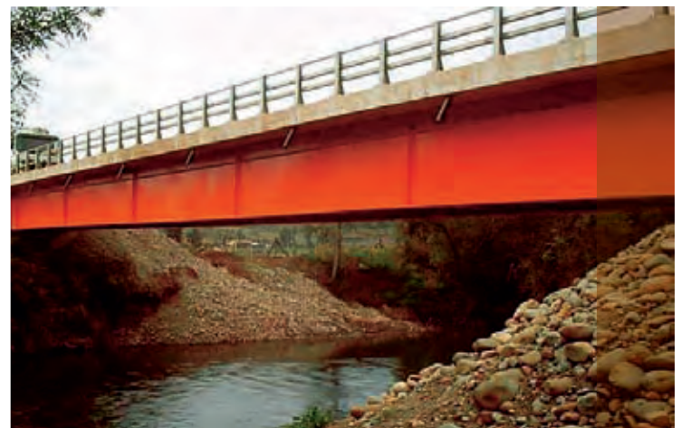
Bridge over the Mulchén River, built by Forestal Mininco as part of the construction work of the bypass towards Mulchén city. This bridge is built with a solid structure of steel beams and concrete paving, fitted out for heavy-traffic.
