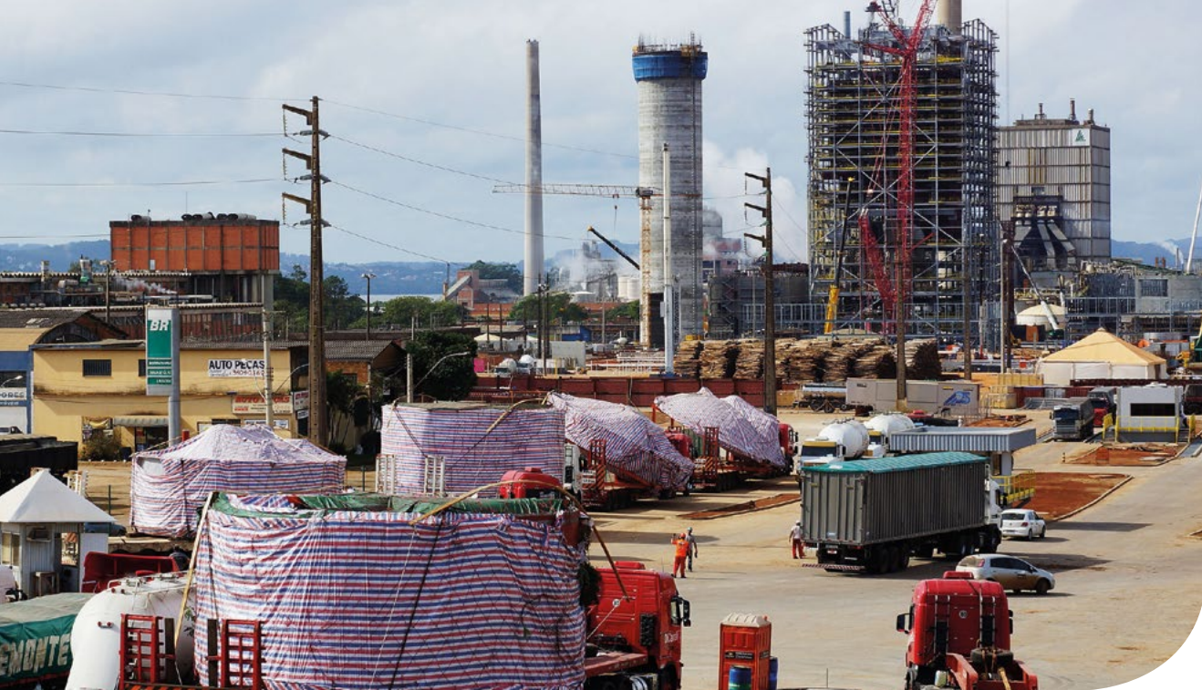
The structure of the recovery boiler, which will be 86 metres high, is already visible.
